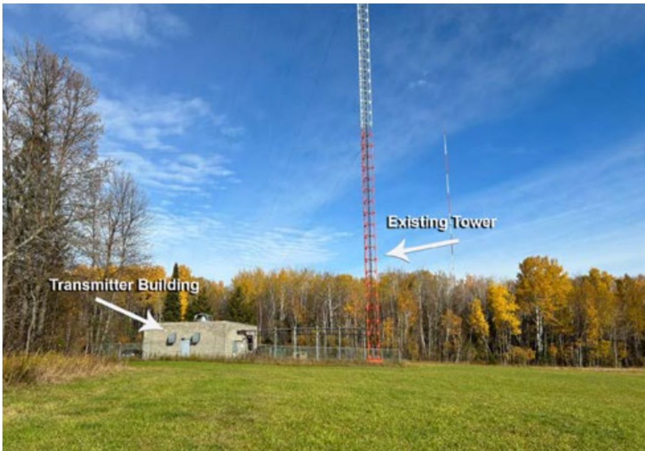
Exhibit 3: Viewshed of Project Site (Showing Existing KAWE Communications Tower, Transmitter Building, and MPR tower in background)
